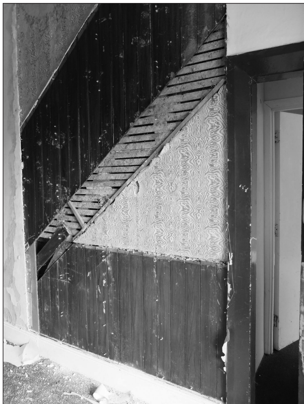
Figure 9. The downstairs hallway after a layer of plasterboard had been stripped back, revealing the outline of the original stairway and timber wainscot. Note that the visible door architrave is a twentieth century addition, probably installed at the same time as the plasterboard.
