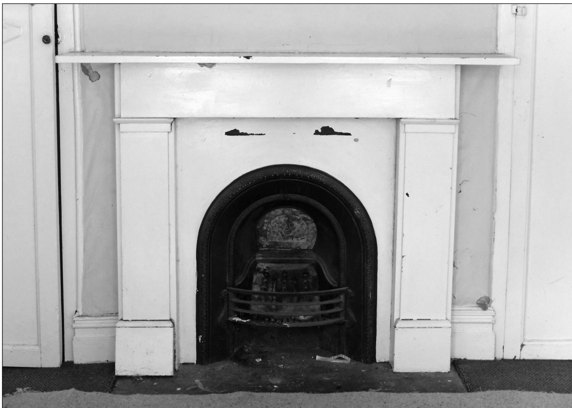
Figure 13. The original black slate fireplace in the south-west upstairs room (Room 3). This had been painted white, but retained its cast iron centre section.
