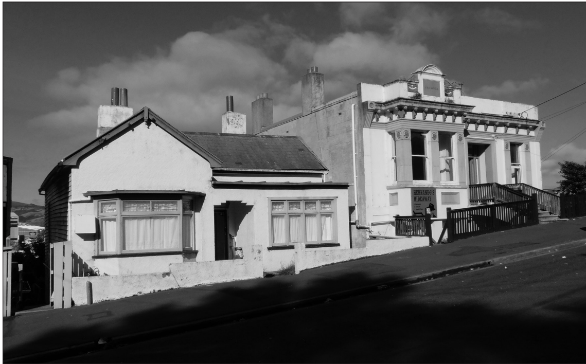
Figure 2. 'Parihaka' at 29 Queen Street on the left, and its neighbour 'Kahanga' on the right at 27 in early 2015.
