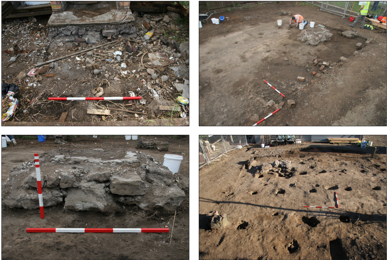
Figure 6. The excavation in progress: top left, modern and historic rubbish and shell midden beneath the leant-to after its removal; top right, the exposed fireplace and chimney foundation, bricks and rubble under the floor in the area around the back door, and scoria rubble under the floor of Room 3; bottom left, fireplace and chimney base showing the plastered hearth surface with layer of levelling midden below on a foundation of irregular scoria rocks; bottom right, the cottage footprint after excavation.
