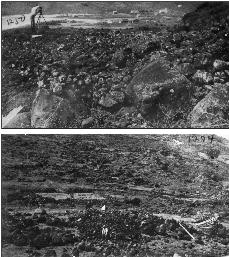
Figure 2. Evidence for Stokes’s surveying methods in photographs. Above: tripod presumably used to support the optical transit (SP 1250; by J.F.G. Stokes, Bishop Museum Archives). Below: white flag used to locate sites from a distance (SP 1274; by J.F.G. Stokes, Bishop Museum Archives).
