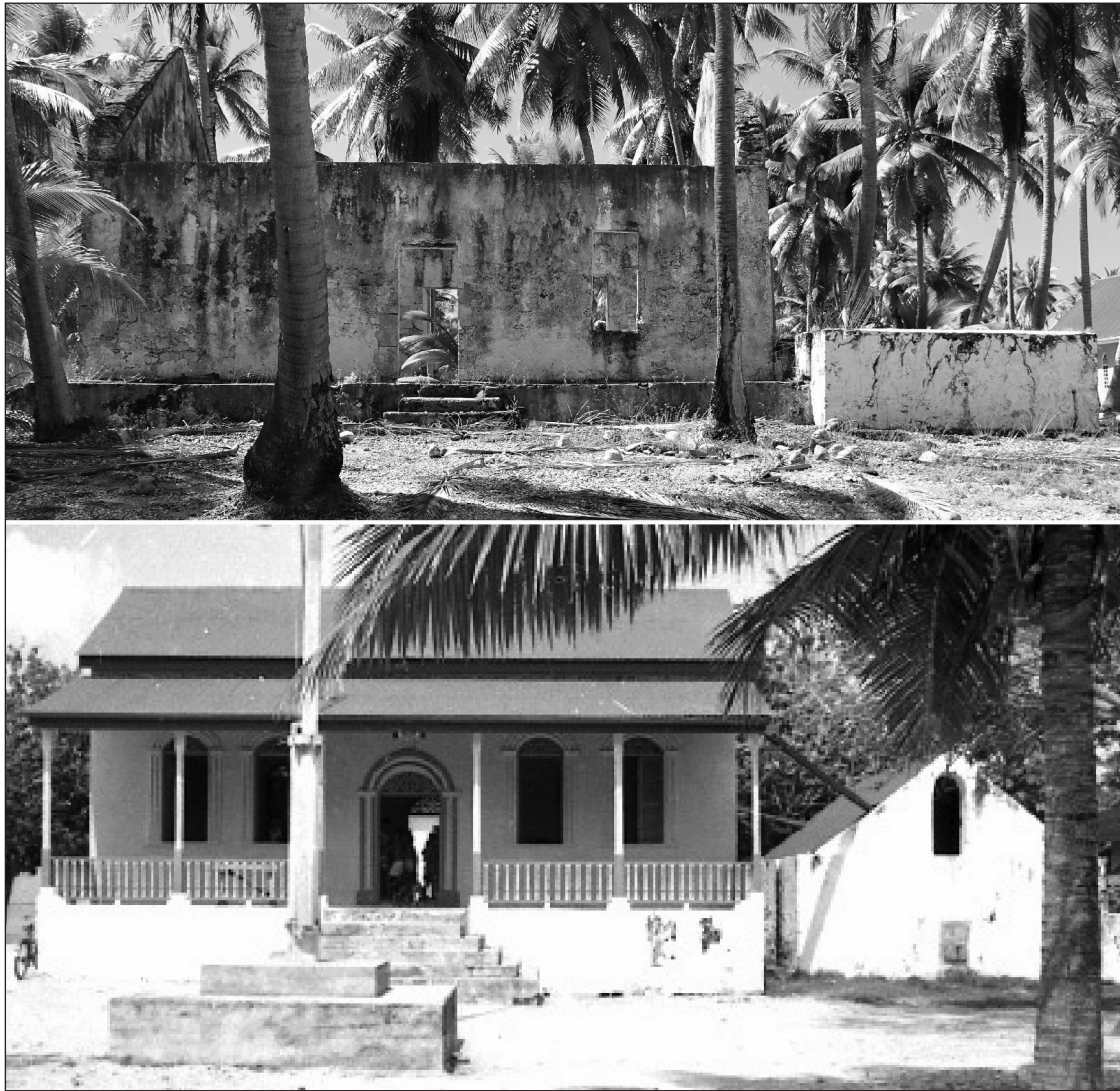
Figure 8. House V'44 with its adjoined cistern, Hokikakika (top); Makemo municipal building, 1967 (bottom), for comparison (source Tahiti Heritage).
