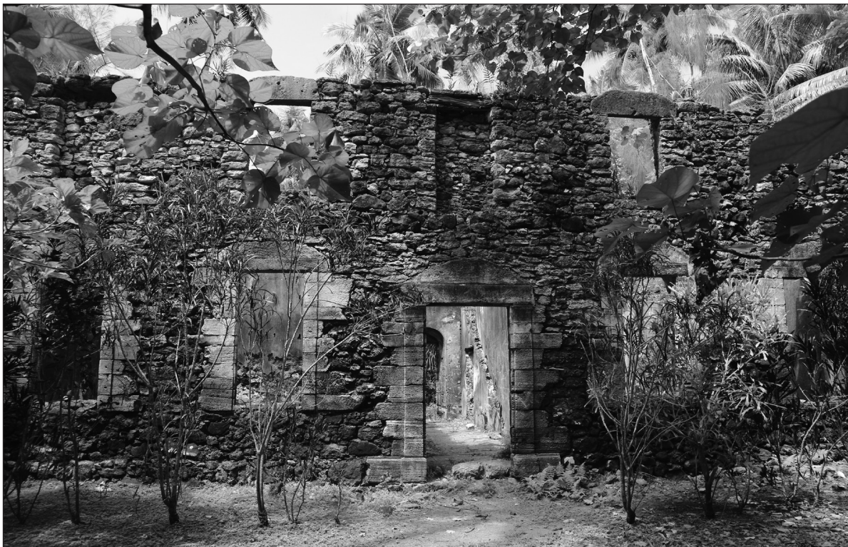
Figure 5. North exterior elevation of the boys' school at Aukena. The diagonal scar in the main hallway is visible on the right hand side, while some of the cabinetry scars in the possible office space are visible in the lefthand ground floor window. The classrooms on the wings are not visible in this photograph.
