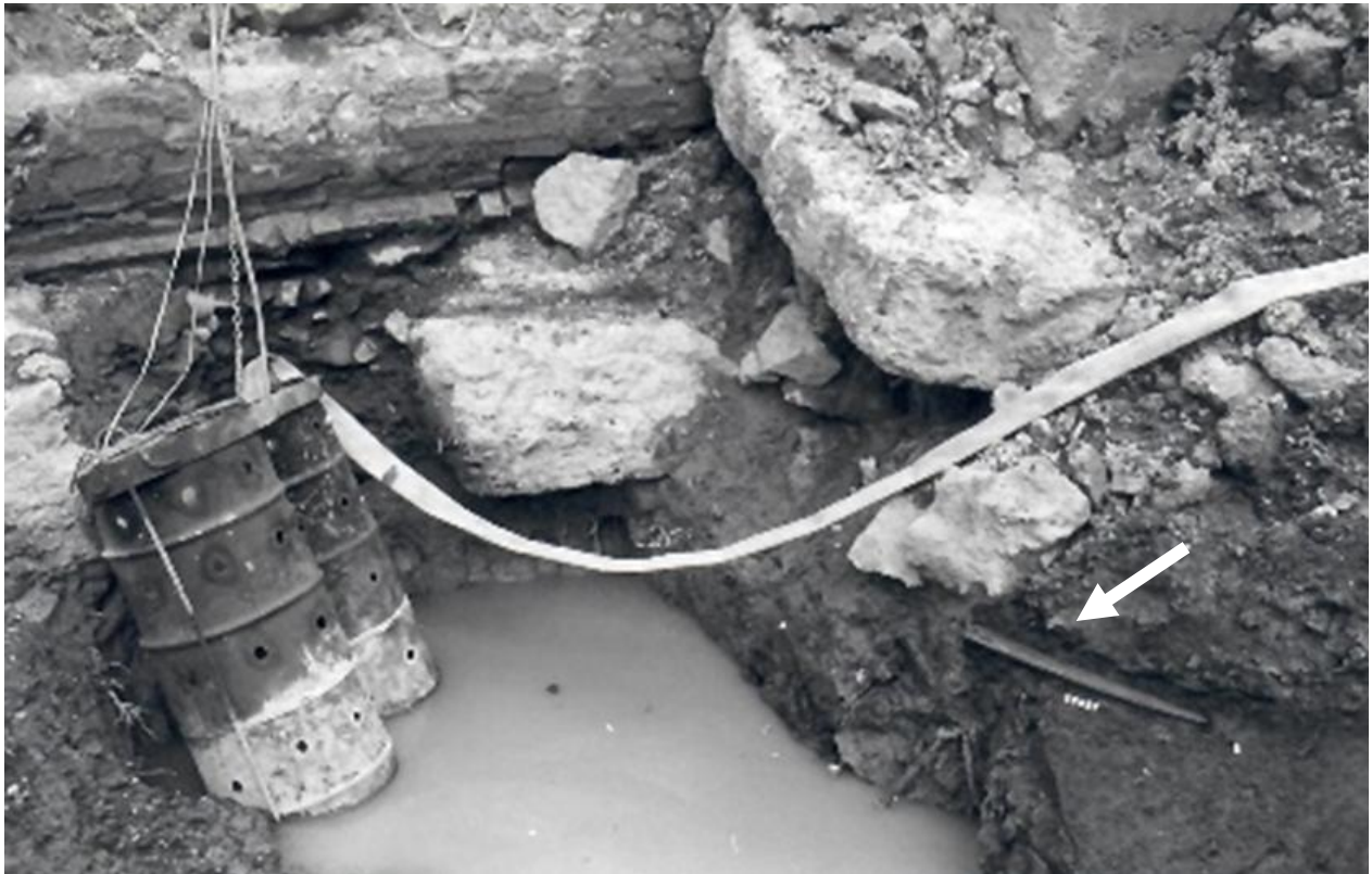
Figure 5: R11/1559 showing sump hole and location of the kō
