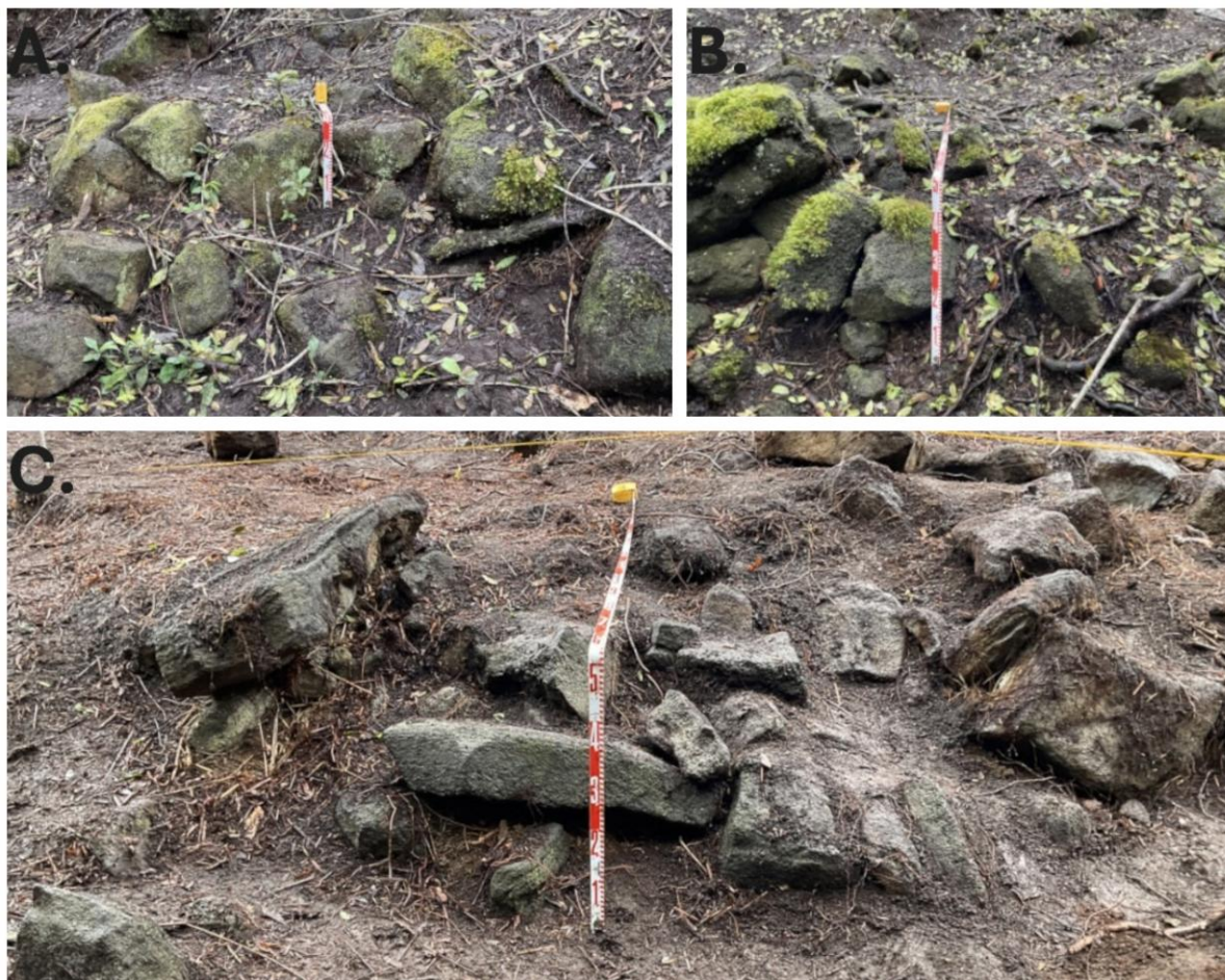
Figure 6: Examples of infrastructure in the gully system. A) is a circular planting pit bounded by 1-2 courses of stone, B) is a small terrace, and C) is a larger terrace. In all cases, infrastructure is roughly stacked and relatively expedient.
