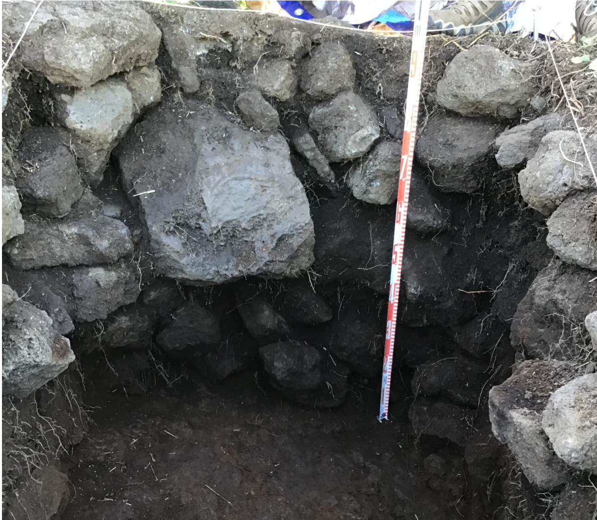
SF10. East wall of T35 of XU30. The date from the feature was taken from beneath the basal course of stone.
