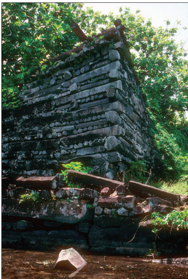
Figure 2. Columnar basalt wall construction using typical header-and-stretcher architectural style. Note use of large boulders as foundation stones. Photo by J.S. Athens.
